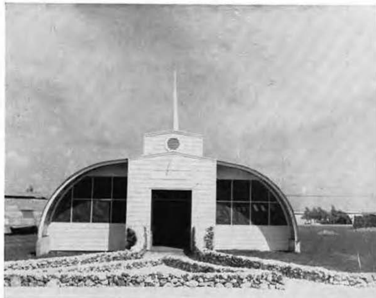
While the heavy equipment men have been pushing the strip, other crews have been busy too. Shops, warehouses, living quarters, a chapel, these too are a vital part of the construction job.
