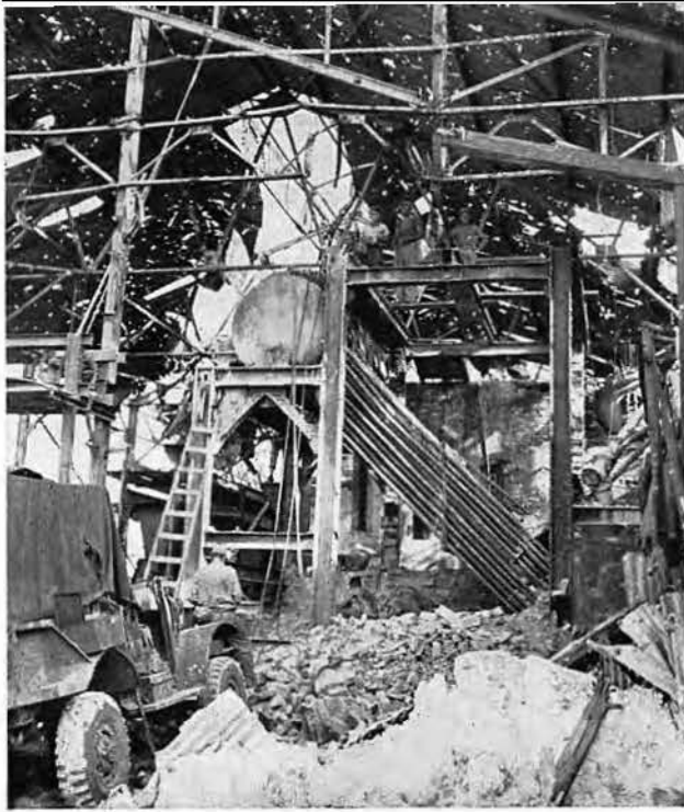
Much valuable material was salvaged from the sugar mill outside Tinian. Here we see the beginnings of the Navy asphalt plant.
