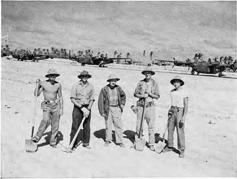
Strip maintenance crew
