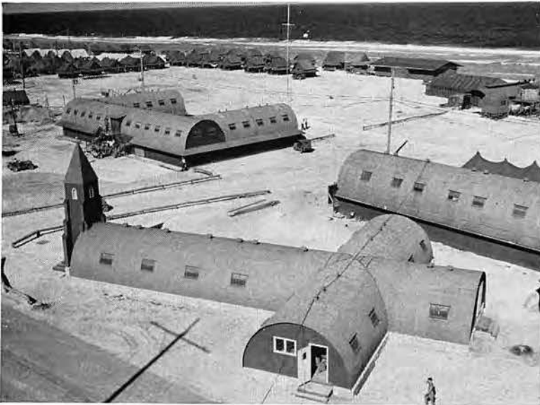
Port Captain's office and signal shack
