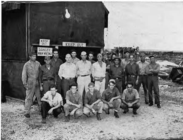
From salvaged Japanese equipment and a minimum of new parts, the electrical crew under Mr. Bigley constructed a modern electrical power plant capable of producing power for a city of 5,000 people.
