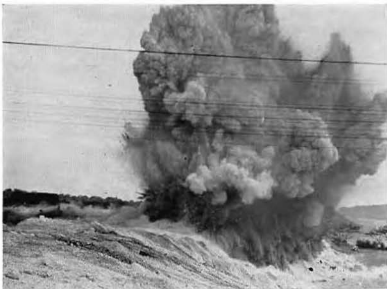
Tons of dynamite and thousands of yards of coral hauled from pits several miles away have affected quite a change. Soon fields, that only a short time ago were covered with sugar cane, begin to look like an air strip.
